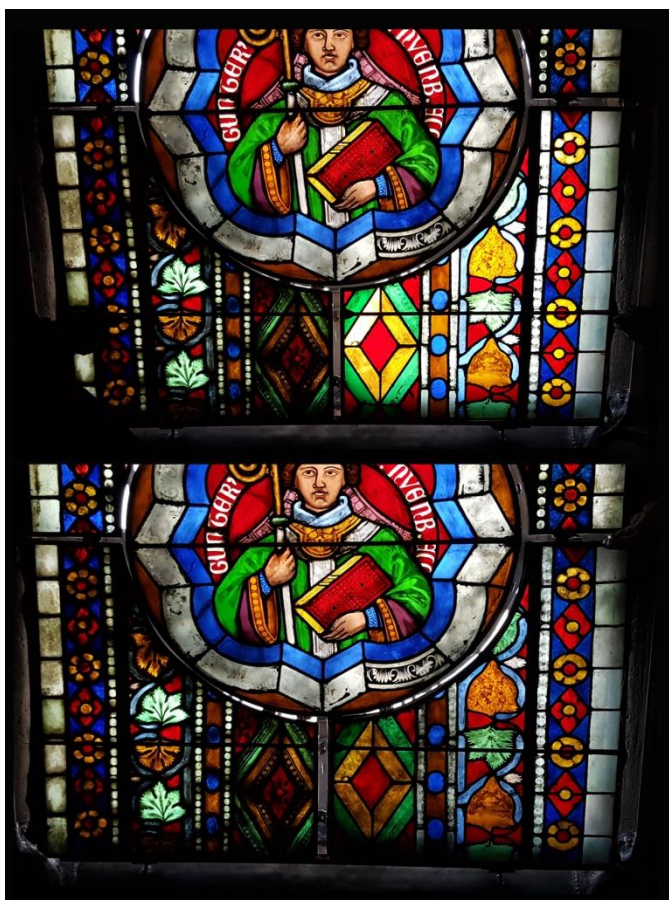
Fig. 2. Naumburg Cathedral: Before and after installation of the darkening plate for panel nwll 1a1.
