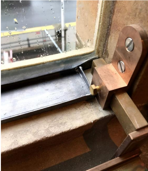
Fig. 1. Lerwick Town Hall, Shetland, west elevation detail showing external glazing, mortar covered with burnt sand mastic "skin", bottom slide bar system placed vertically on stone cill, the leg extension to accommodate any overall height changes, and the lead condensate tray, 2017. © Cannon-MacInnes.
