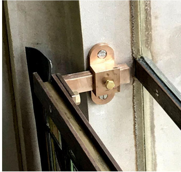
Fig. 2. Lerwick Town Hall, Shetland, west elevation detail showing external glazing, mortar covered with burnt sand mastic "skin", vertical slide bar system placed vertically on new stone mullion, the manganse bronze support bar, and a fully conserved "middle" panel in place, 2017. © Cannon-MacInnes.
