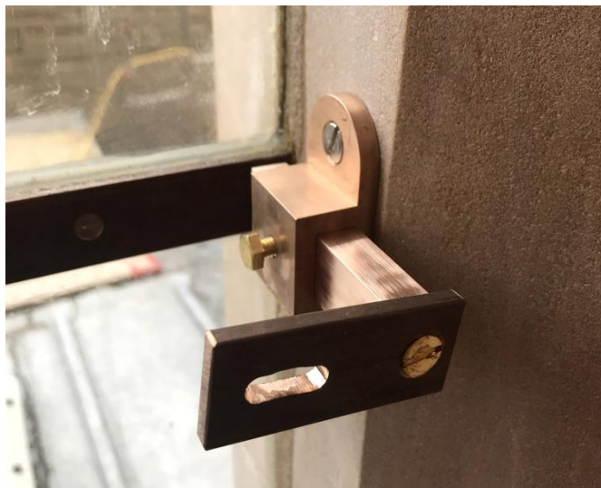
Fig. 4. Lerwick Town Hall, Shetland, south elevation detail showing the internal slide bar, which allows the whole system to be finely tuned to fit perfectly. Each panel can be adjusted on site, slightly up, down, in, out, right or left, 2017. © Cannon-MacInnes.
