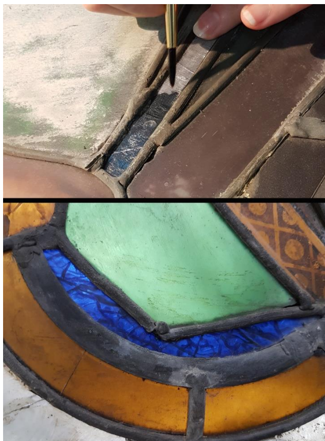
Fig.3. Craquelé consolidation technique and post treatment result in nwIII 2a © Vereinigte Domstifter.
